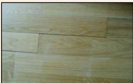
Excessive Gapping
